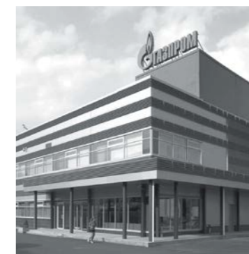
СК «Газпром Прометей» Construction Company "Gazprom Prometheus"
